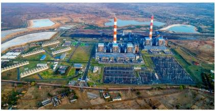
The power plant supplied 4620 Mega Watts of energy. Out of these 2000 is supplied to HARYANA, 2000 to GUJARAT government, & 620 is internally used. It uses HVDC (High Voltage DC) for transmission to HARYANA as it is a long distance transmission it is to be converted into DC first & then it is again recovered. Live status of frequency and power generated was available in the control room.
